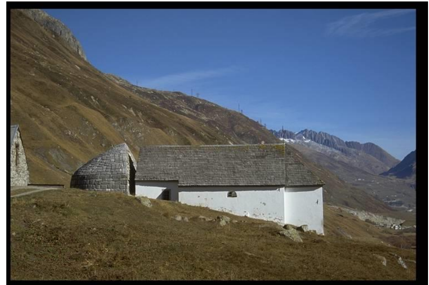
Passive defense structure
