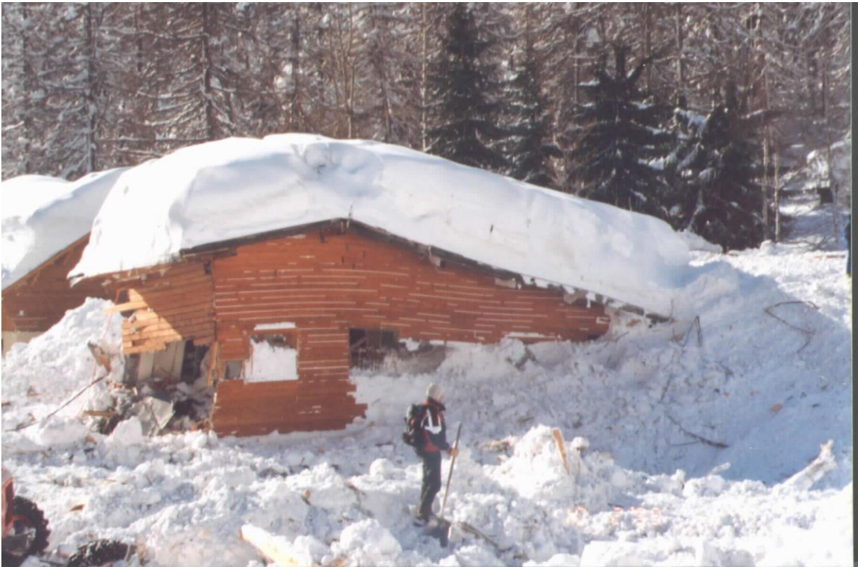
Montroc (Haute Savoie, France), 9 February 1999, building moved and destroyed
