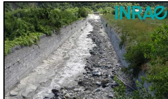
Saint Bernart torrent (France)
